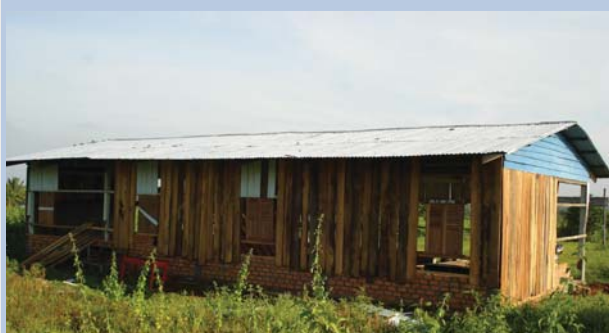
Chub korki Primary School in delay for contruction
